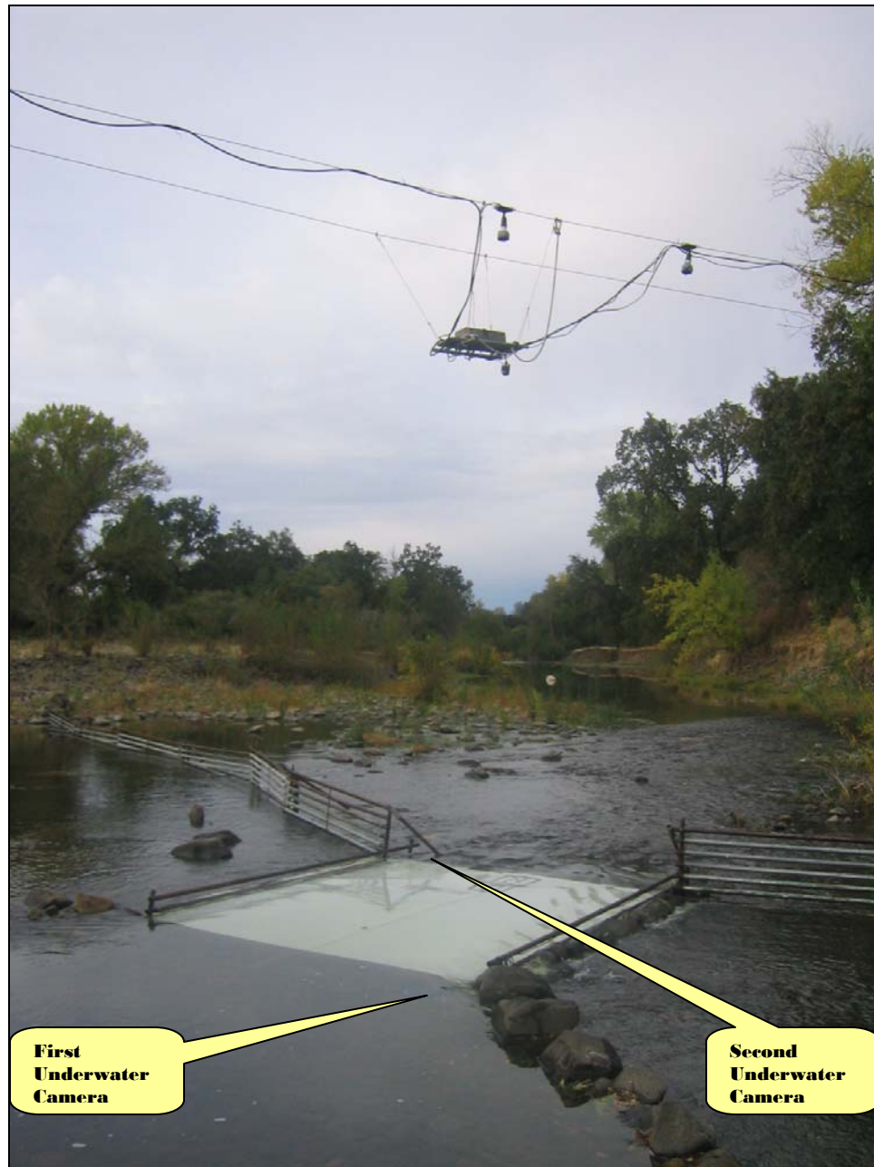
Figure 3. Camera box suspended over Bear Creek at a height of about 12-feet (3.6 m) from the water's surface using a two main cable system constructed of 5/16-inch (7.9 mm) galvanized steel cables. Also showing the location of the two underwater cameras and the weir opening allowing fish passage.
